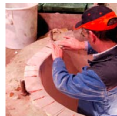
Before inserting the Dorit prefabricated crucible, first install the insulation and the floor-molded bed for the crucible.
