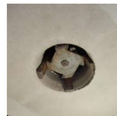
Lifting device without steel bottom plate
